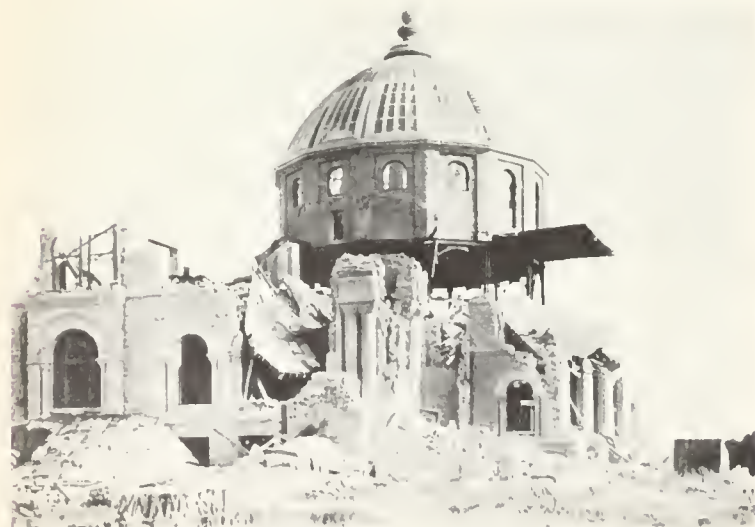
FIG. 8. Library at Stanford University after the 1906 earthquake. The steel supported rotunda was relatively undamaged, but the unreinforced masonry collapsed. Photo from the J. C. Branner collection, courtesy Stanford University.
