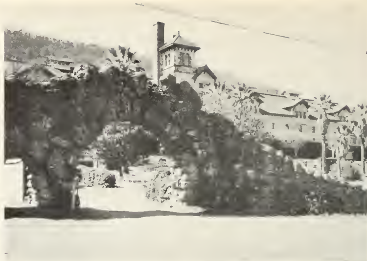
FIG. 2. Cresta Blanca Winery, north of St. Helena, Napa County. Constructed in 1889 of dacite and rhyolite blocks.
