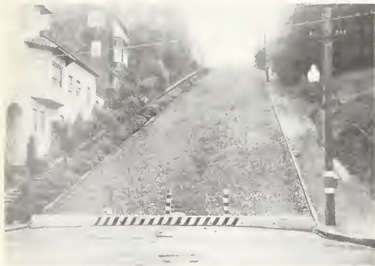
FIG. 8. Baker Street, San Francisco. Looking south from Vallejo Street. Pavement made of basaltic paving cobbles. Photo courtesy Bureau of Engineering, City and County of San Francisco.
