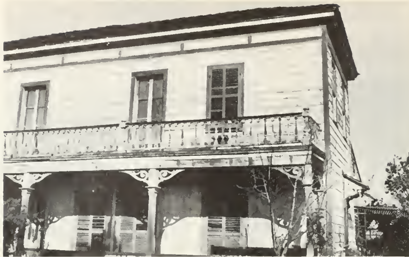
FIG. 9. Frame house covering two old adobes at 770 Lincoln Street, San Jose. Original adobes built in the late 1830's and early 1840's. Photo by Mary Rae Hill.
