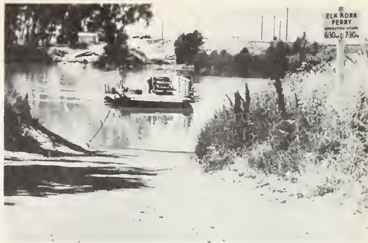
FIG. 32. Elkhorn Ferry, near Woodland, Yolo County, one of the few ferries operated by the State Highway Department. Ferry carries three cars. An upstream cable holds the boat on its course and the ferry is moved by cables and a power winch. Photo courtesy San Francisco Chronicle.
