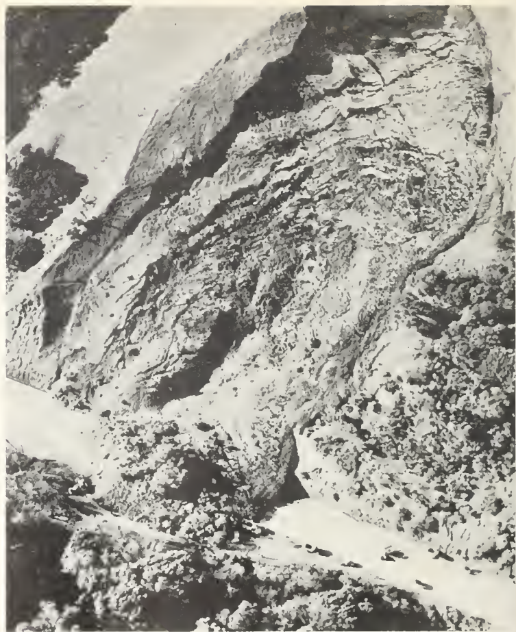
FIG. 33. The landslide of December 9, 1950, on Tunnel Road (State Highway 24) between Oakland and Orinda. Trees brought down in the slide and the earth moving equipment in the right foreground give some idea of the magnitude of the slide. Rock exposed in the road cut in the extreme left center of the picture is steeply west-dipping basalt of the Moraga volcanic series; rock to the right of the toe of the slide is gently east-dipping gravel and sand, probably part of the Orinda formation. Slide material was principally clay and gravel but some basalt came down too. The slide is at the axis of a faulted anticline. The State Highway Department spent almost seven months removing the slide from highway and hillside and placing drainpipes to reduce chances of another slide. The highway was almost completely blocked for several days and the temporary by-pass was a bottleneck on the heavily travelled highway for many months afterward. Photo by Bill Young, courtesy San Francisco Chronicle.
