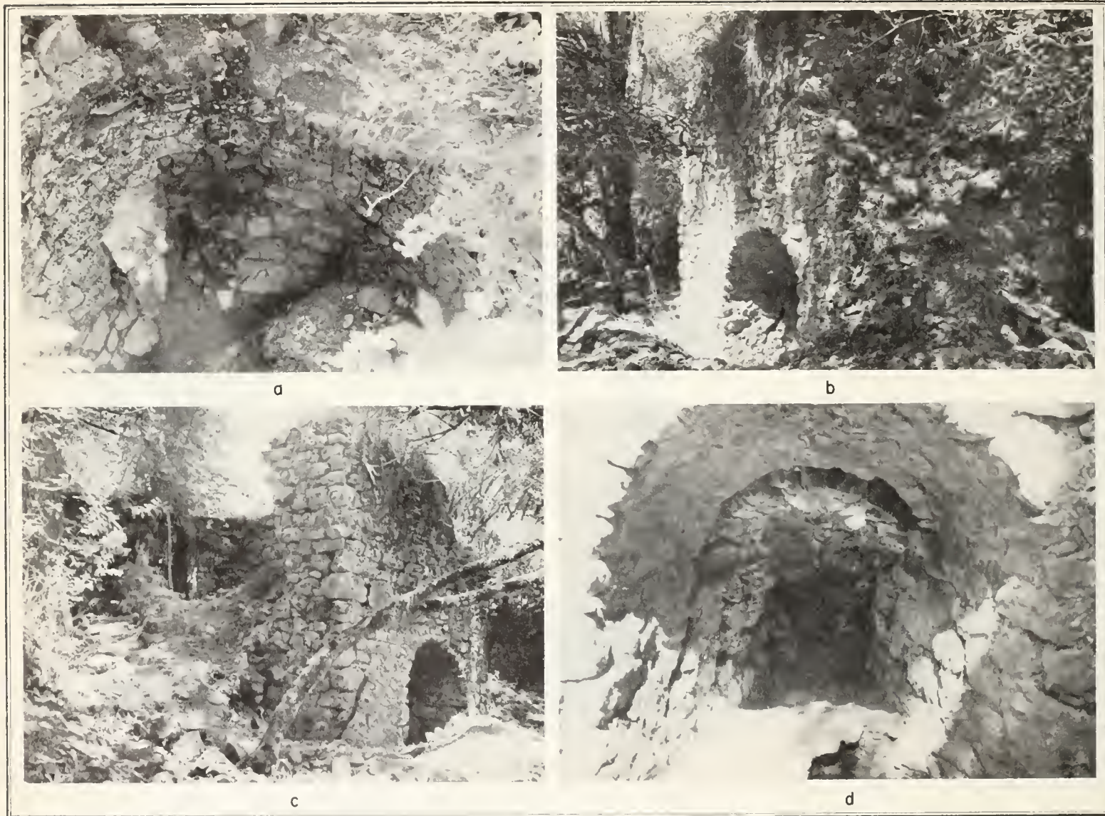
FIG. 3. Photographs showing kiln 2. a , Inside of kiln, showing inner casing and fire arch; mason work has been carefully done. b , c , Outer casing and fire arch. Stone masonry on outside casing proved resistant to weathering, but inside chunky "fill" is crumbled and slumped. d , Front view of fire arch and grate; floor (grate) is composed of 8-inch layer of rock set in mortar or fire clay. Photos by J. Quast.
