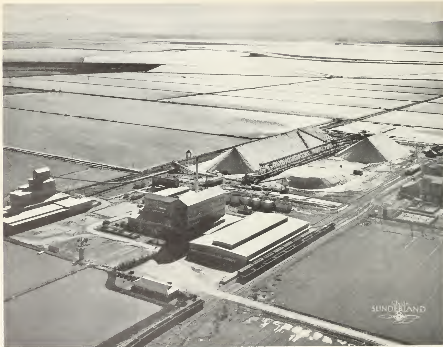
FIG. 1. Newark, Alameda County, plant of Leslie Salt Company. Bay water is concentrated by solar evaporation in the large irregular ponds in the distance and then run into small rectangular ponds in the middle distance where salt precipitates. The crude salt is then scraped up, washed with brine to remove some impurities and stock piled in the long stacks seen in the right middle ground. The washing plant is behind the stock piles. Crude salt then passes through the processing plant to the left of the stock piles where it is either loaded directly into railroad cars or trucks for outside delivery or ground, sized, and sacked. A portion of the crude salt is refined by re-solution and vacuum evaporation in the building in center of the picture. Part of the Morton Salt Company refinery is visible at the extreme right of the picture. Crude salt refined in this plant is purchased from Leslie Salt Company. Photo by Clyde Sunderland, Oakland.
