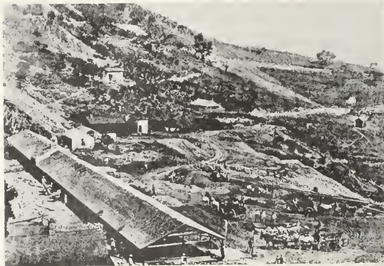
FIG. 4. New Almaden in the early 1860s. Opening of the main tunnel is in the left middle distance. The shed and large level area to the right of it were used to stack and sort ore coming from the tunnel. These level cleaning grounds were called planillas by the Mexicans. Compare this photo with Figure 1, taken in the same direction at a much later date. Photo of an old drawing, courtesy Jimmy Schneider, San Jose.
