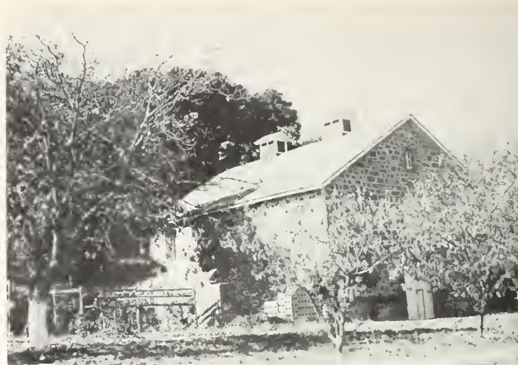
FIG. 7. Holt wine cellar on Holt Ranch, east of St. Helena, Napa County. Constructed in 1896 of perlite rock from quarry near site of cellar. Photo by G. D. Hanna.
