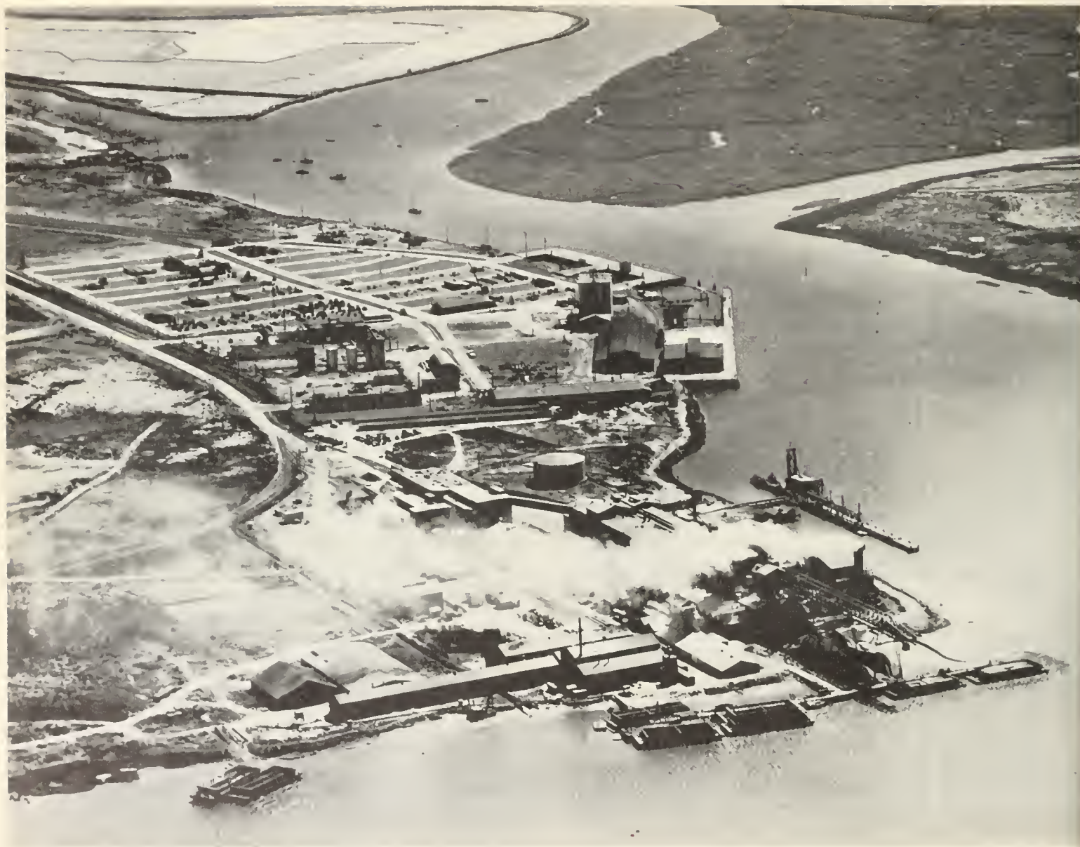
FIG. 1. Pacific Portland Cement Company's Redwood City plant, the only one in California using oyster shells and bay mud as the basic raw materials for cement manufacture. Photo by Fred Mac Acro Photos, courtesy San Francisco Chamber of Commerce.
