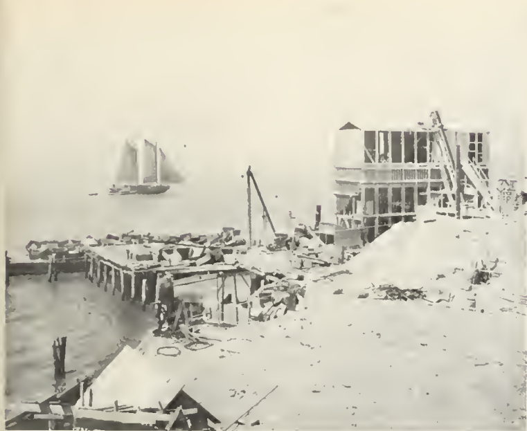
FIG. 2. An old photograph of the Healy-Tibbetts rock quarry crushing plant and loading dock near Winehaven, west of Richmond, Contra Costa County. Crushed rock once was shipped by barge in large open boxes as shown in the left middle ground. Quarry was in sandstone of the Franciscan formation. Site is now occupied by installations connected with the Standard Oil Company refinery at Richmond. Photo courtesy Pacific Gas and Electric Company.
