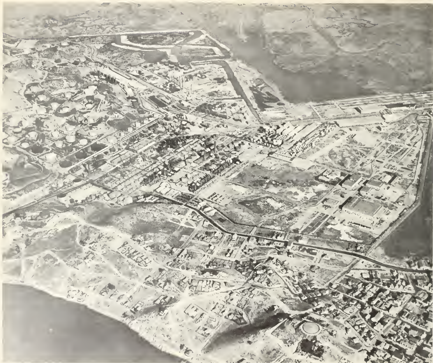
FIG. 2. Richmond oil refinery of Standard Oil Company of California, showing the numerous storage tanks which serve the refinery. Point San Pablo is to the left of the area shown in the photograph; City of Richmond to the right. Photo by Commercial Photo and View Company, courtesy Contra Costa County Development Association and San Francisco Chamber of Commerce.
