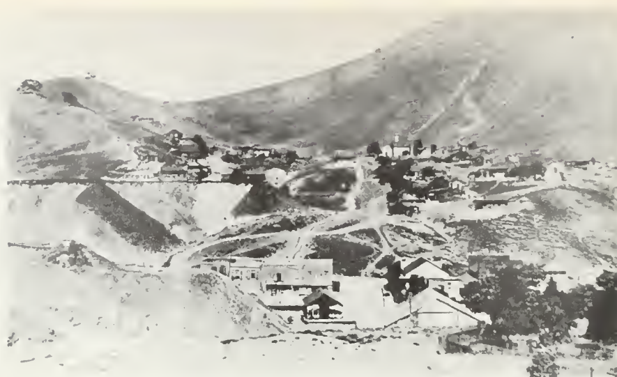
FIG. 41. Nortonville in the late 1870s, camera facing west across School Hill. Steepled building at the foot of the hill in the right middle ground is Nortonville Grammar School. The extensive mine dumps and trackways leading to them from the Black Diamond mine are prominent in the left foreground. Photo courtesy W. F. Jones, San Francisco.
