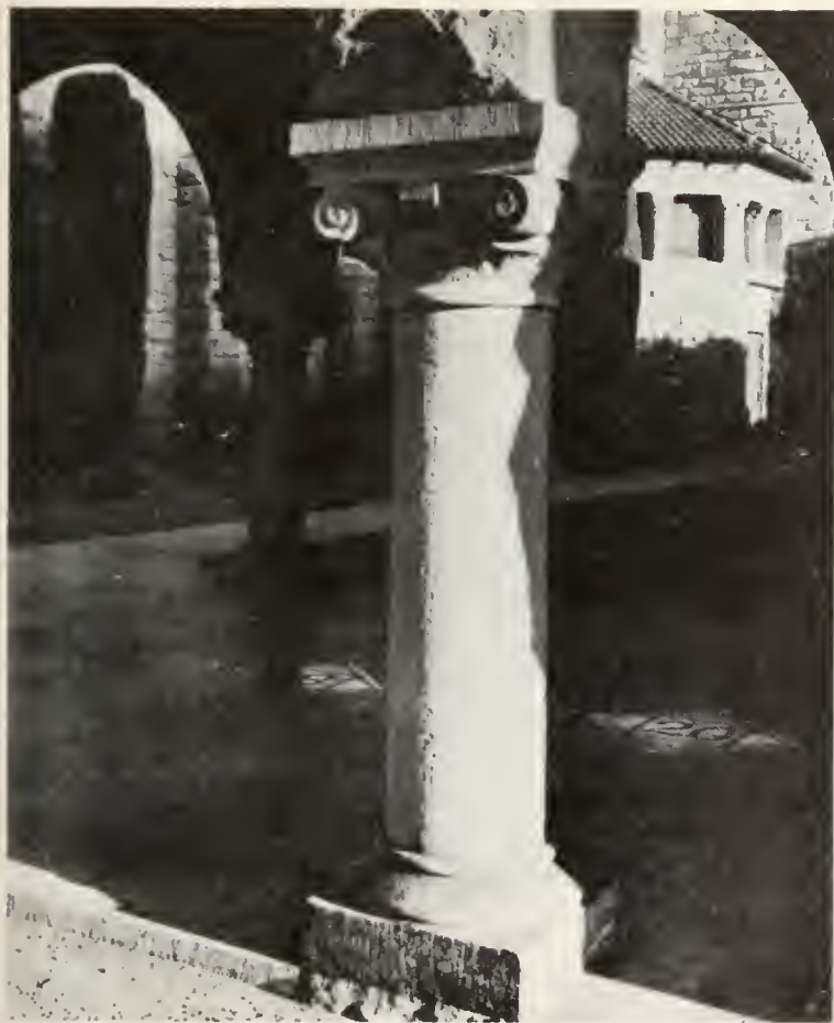
FIG. 2. Detail of stone construction on the Stanford campus. Rock used is Upper Cretaceous sandstone from Graystone Station quarry located nine miles southwest of San Jose. Photo courtesy of Stanford University.
