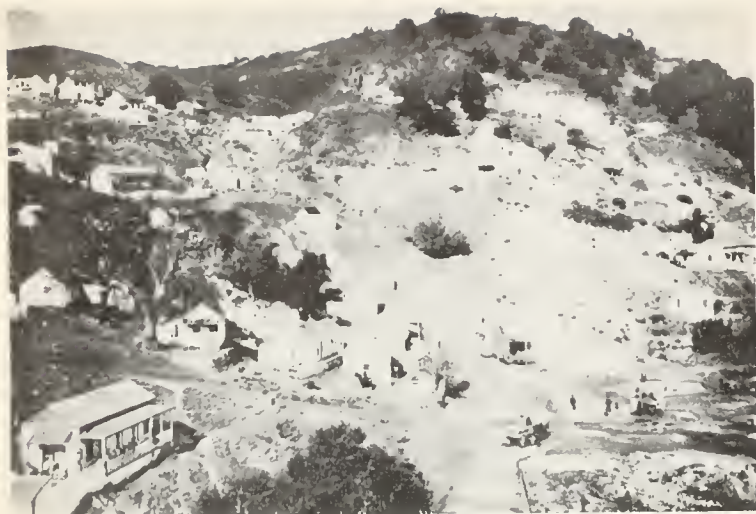
FIG. 1. An old photo of the southeast slope of Mine Hill, New Almaden, Santa Clara County, showing the lower section of the Mexican camp. The level area in the right foreground is a planilla or ore-cleaning ground. Photo courtesy Jimmie Schneider, San Jose.
