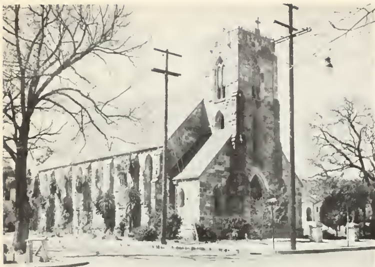
FIG. 1. St. Helena Church, St. Helena, Napa County. Constructed in 1879 of rhyolite, andesite, and dacite.
