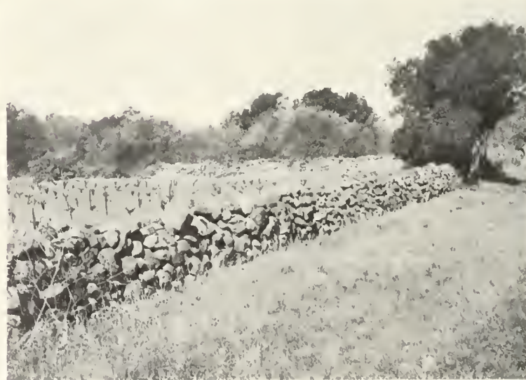
FIG. 4. Stone fence on Silverado Trail, east of Yountville, Napa County. Built of field boulders of andesite, rhyolite, and basalt.
