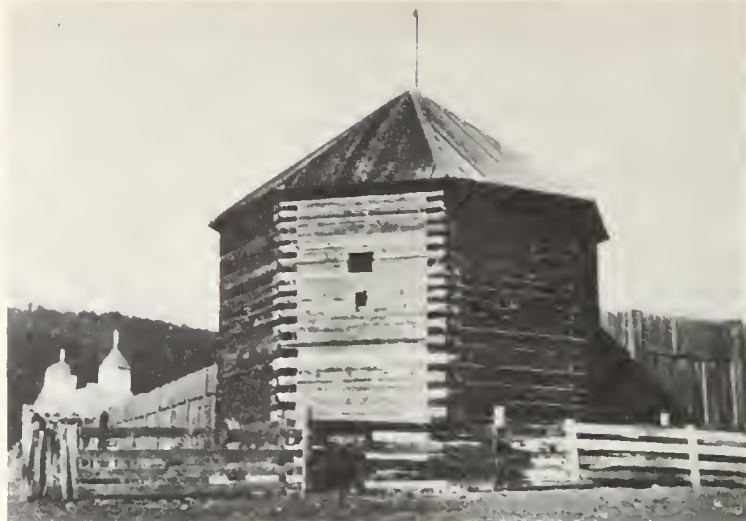
FIG. 10. Detail of one of the restored blockhouses at Fort Ross, showing cannon ports and massive timber construction. Spires of the restored Greek Orthodox Church at extreme right.
