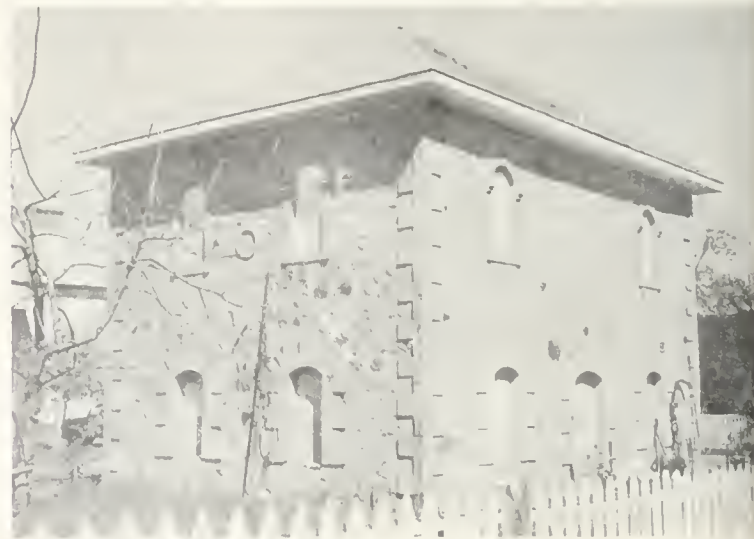
FIG. 9. Old St. Helena Winery, St. Helena, Napa County. Built in 1880 of rhyolite, andesite, and dacite.
