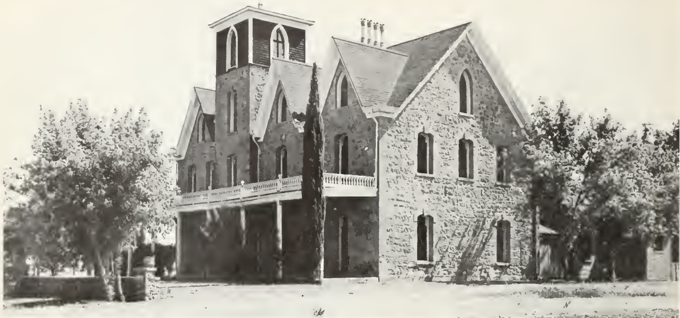
FIG. 6. The stone mansion built by John Marsh in 1855 still stands close to the Marsh Creek road a few miles south of Brentwood, Contra Costa County. Photo courtesy of Pacific Gas and Electric Company.
