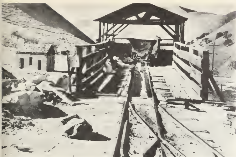
FIG. 1. Silica-sand loading platform at the site of the old coal mining town of Nortonville northeast of Mount Diablo, Contra Costa County. Eocene rocks of the Nortonville-Somersville area, important in the 1880s for their coal veins, have since been mined intermittently for quartz sand for use in glass or refractories. Neither the sandstone nor the coal veins have been exhausted, but remain as potential sources of mineral wealth. Photo by Bob Campbell, April 1947, reproduced courtesy San Francisco Chronicle.
