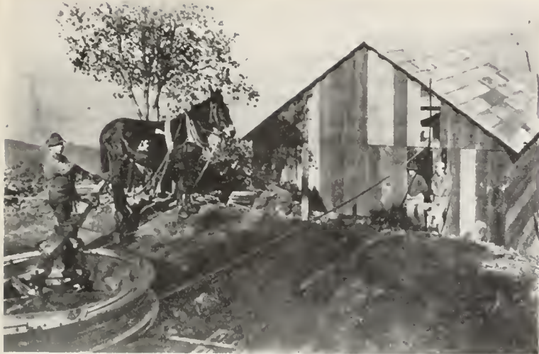
FIG. 5. Mule-driven windlass for hoisting and lowering the skip (shaft car) in the prospect Shaft No. 1 at New Almaden, 1880. Photo courtesy Jimmie Schneider, San Jose.
