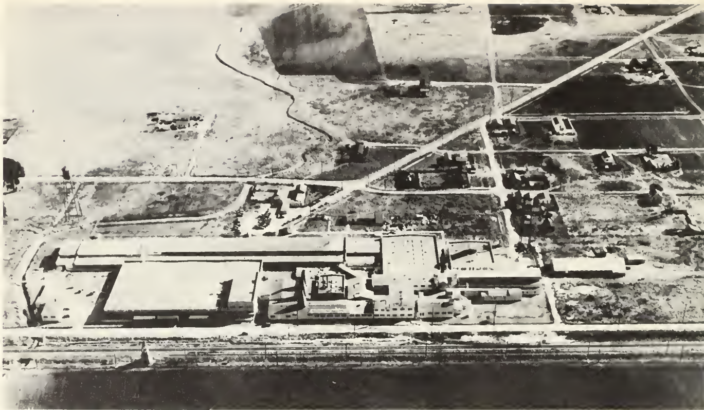
FIG. 4. Standard Sanitary Manufacturing Company plant at Richmond, Contra Costa County, manufacturers of all types of sanitary ware. Photo by Commercial Photo and View Company, courtesy San Francisco Chronicle.
