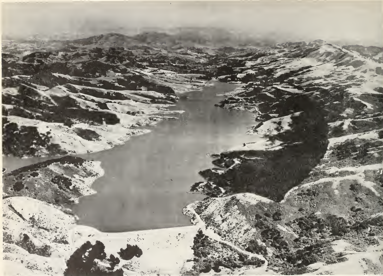
FIG. 1. San Pablo reservoir in San Pablo Canyon east of Berkeley and north of Orinda. Largest of the four water-storage basins for the East Bay Municipal Utility District, the reservoir has a capacity of 14 billion gallons. Water for the reservoir comes from the Mokelumne River in the Sierra Nevada. Hills on either side of the reservoir are principally land-laid sediments and interbedded lava flows of Pliocene age. Photo by Commercial Photo and View Company, courtesy East Bay Municipal Utility District.
