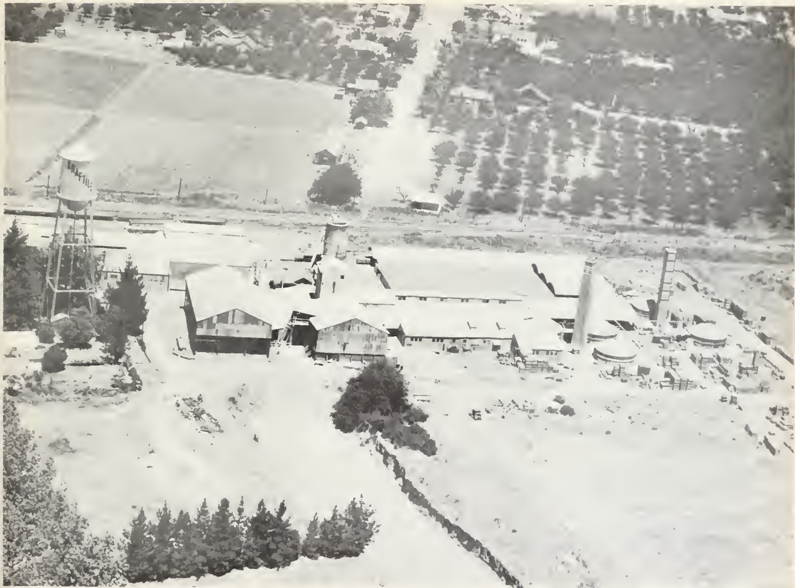
FIG. 2. Ceramic ware plant of Krafftile Company two miles northwest of Niles, Alameda County. Glazed structural units, patio tile, and various kinds of special brick are the principal products. Plant consumes local alluvial clay and light burning clays brought from Lincoln, Placer County. Photo by Fred Mac, courtesy Krafftile Company.
