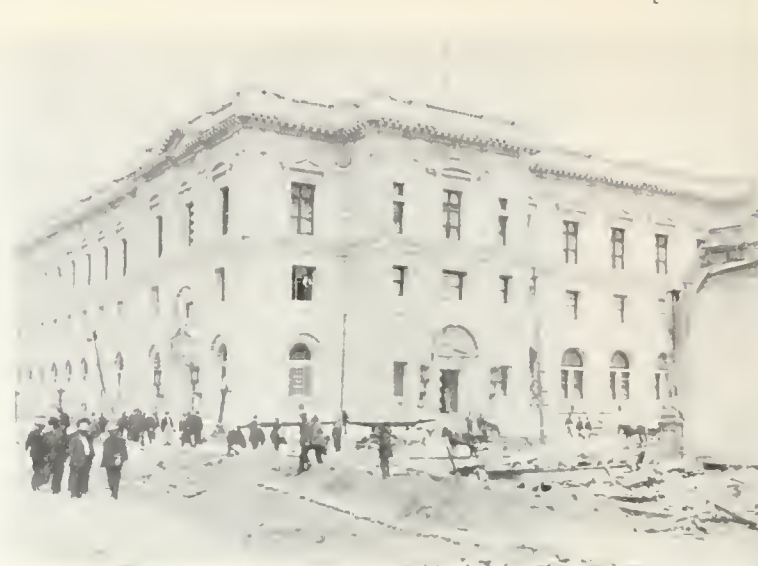
FIG. 7. San Francisco Post Office at Mission and Seventh Streets after the 1906 earthquake, showing that buildings can be designed that can withstand severe earthquakes. Most of the older buildings in the vicinity were demolished.
