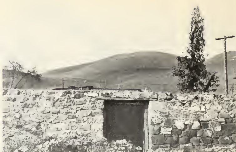
FIG. 6. Foundation of Vallejo flour mill, located just east of the Highway 17 underpass at Niles. Building was completed in 1856. Photo by Mary Rae Hill.
