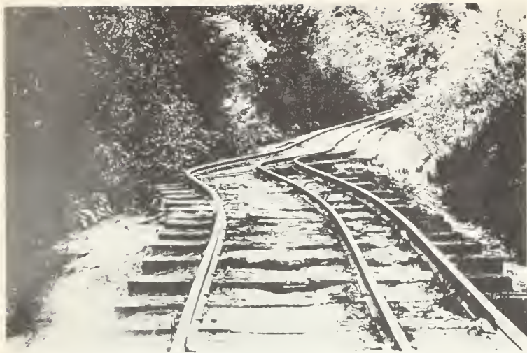
FIG. 11. Old railroad which ran between Los Gatos and Santa Cruz, badly warped at the point of intersection with the San Andreas fault break of 1906. Photo from the J. C. Branner collection, courtesy Stanford University.
