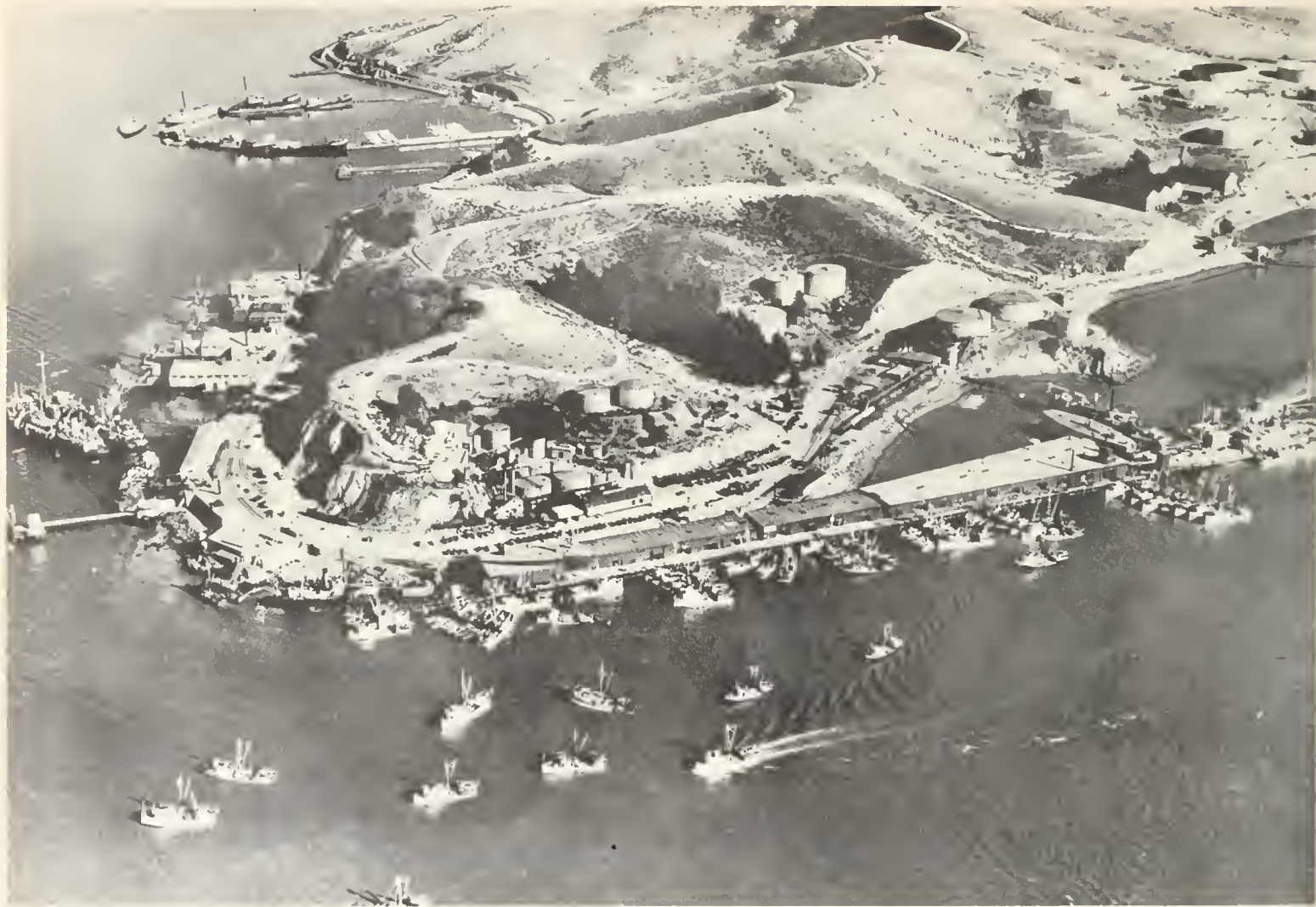
FIG. 1. Oil storage and dock-loading facilities at Point San Pablo near Richmond, California, part of the transportation facilities serving the Richmond oil refinery shown in Figure 2. Photo by Commercial Photo and View Company, courtesy San Francisco Chamber of Commerce.
