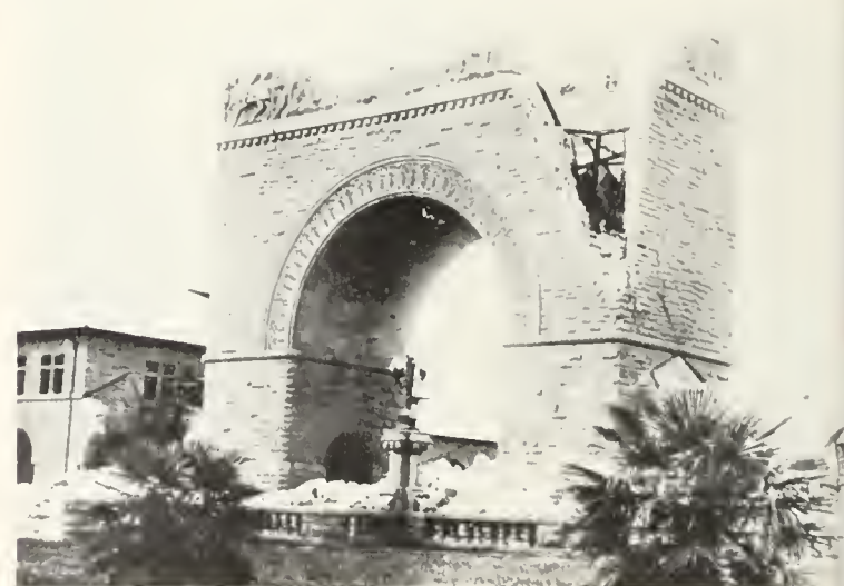
FIG. 9. Memorial Arch on the Stanford campus, damaged in the 1906 earthquake. The basal pillars of the structure were restored afterward, but the damaged arch was removed. Photo from the J. C. Branner collection, courtesy Stanford University.
