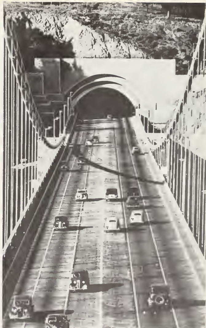
FIG. 28. West entrance to Yerba Buena Island tunnel on the San Francisco-Oakland Bay Bridge, photographed about 1938. Rocks above the concrete portal are sandstone of the Upper Jurassic Franciscan formation. The sandstone and shale of Yerba Buena Island, through which the tunnel was driven, did not prove strong enough to support themselves while such a large opening was being driven, so a narrow arch-shaped slice was first taken out and ceiling supports were put in as the driving of the tunnel progressed. Photo courtesy California Toll Bridge Authority and San Francisco Chronicle.
