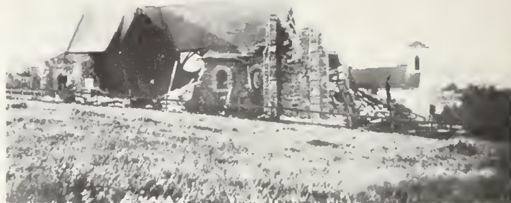
FIG. 4. Old stone church at Tomales damaged by the earthquake of April 18, 1906. Photo from J. C. Branner collection, courtesy Stanford University.
