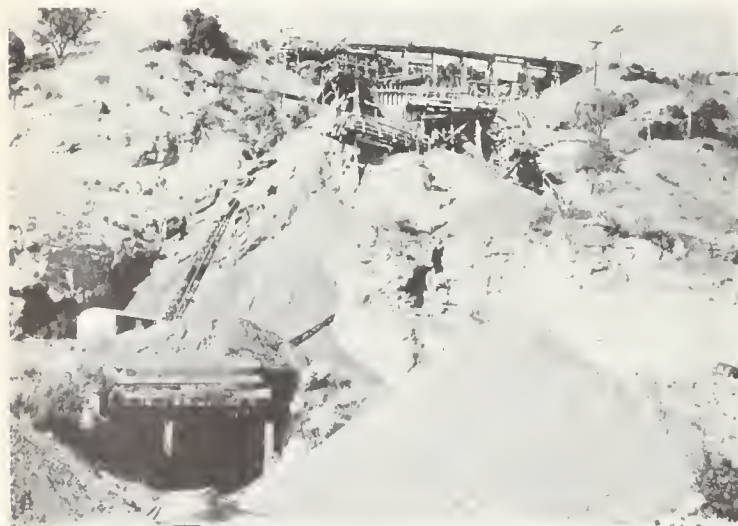
FIG. 12. J. M. Nelson quarry, near Cordelia, Solano County. General view of crushing and screening plant and stock pile of crushed basalt.
