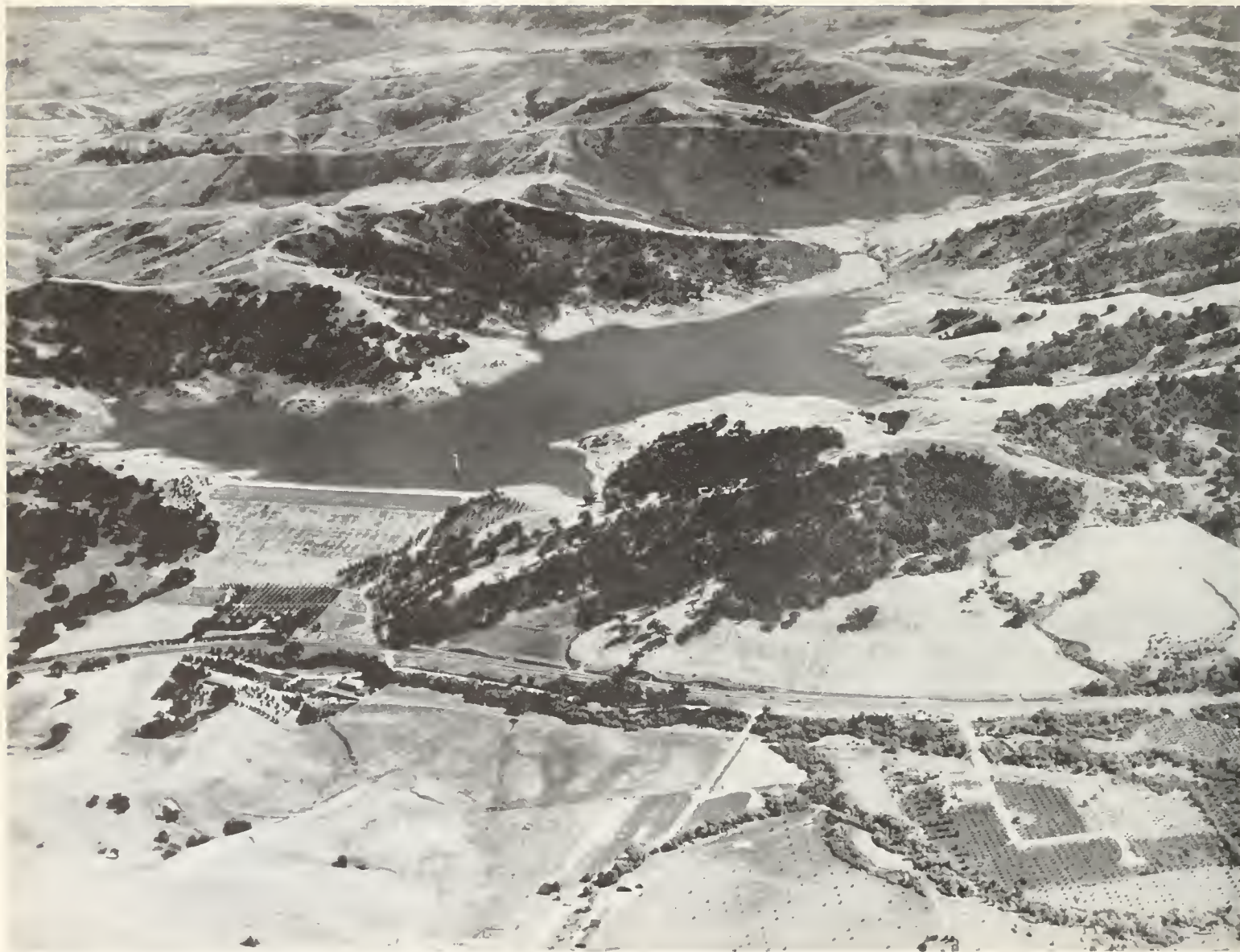
FIG. 2. Lafayette reservoir in the hills southwest of Lafayette, Contra Costa County. Completed in 1932, it is the smallest of the four storage basins that impound the water brought in by aqueduct from the Mokelumne River in the Sierran foothills. It has a capacity of 1\frac{1}{2} billion gallons. Ridges in the middle distance are soft land-laid clays and poorly consolidated sands and gravels of Pliocene age. Photo by Commercial Photo and View Company, courtesy East Bay Municipal Utility District.
