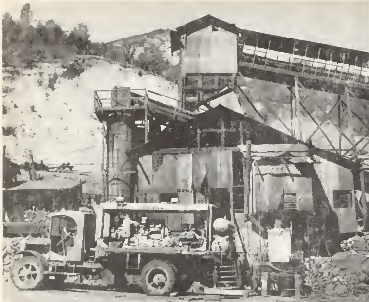
FIG. 1. Part of the mill at Mount Diablo quicksilver mine, located four miles southeast of Clayton, Contra Costa County. The large condenser tubes are a conspicuous part of most quicksilver refining mills.
