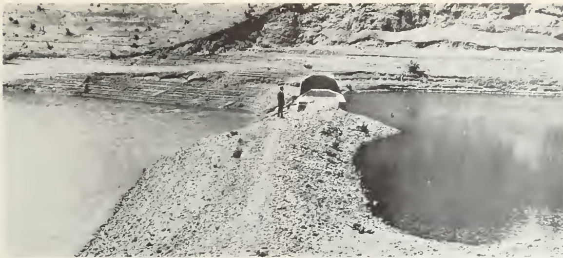
FIG. 5. Rock and earth dam between Upper and Lower Crystal Springs Lakes was offset but not disrupted by the San Andreas fault movement of 1906. Damage is no longer visible.
