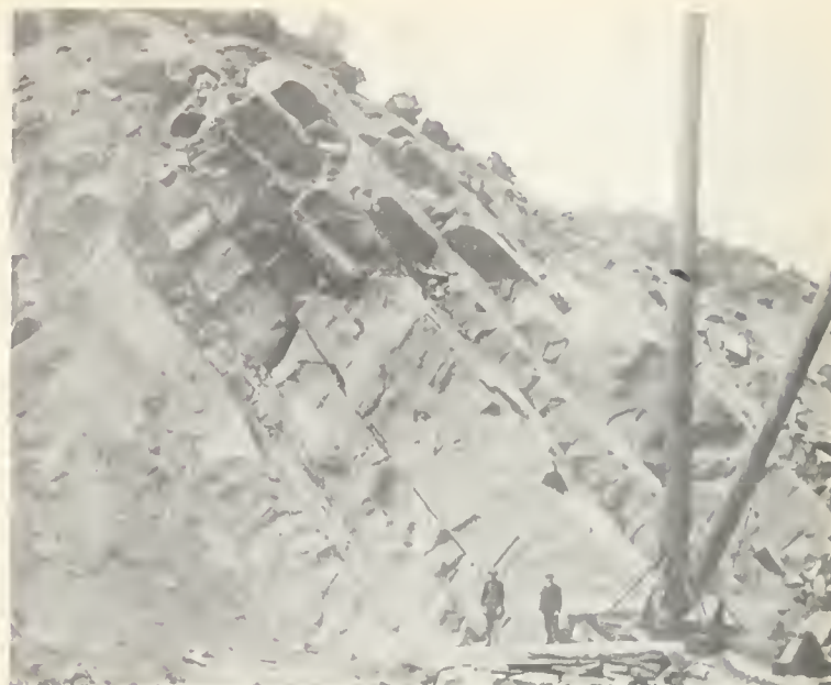
FIG. 3. Colusa sandstone quarry near Sites, Colusa County, from which building stone for such San Francisco structures as the Ferry Building, St. Francis Hotel, and Flood Building was taken. Sandstone beds of Upper Cretaceous age range from 18 inches to 35 feet in thickness. Photo courtesy Pacific Gas and Electric Company.
