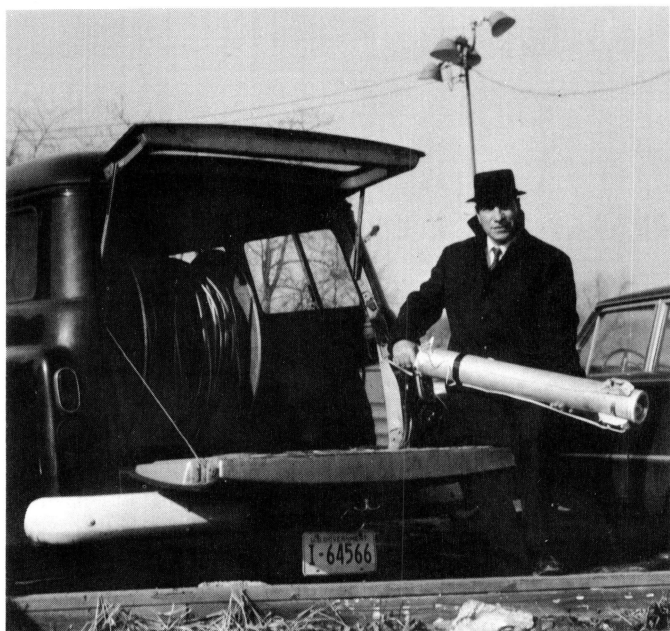
FIGURE 172.1.—Camera with attached lights. A reel, wound with 1,300 feet of 24-conductor cable, is mounted in the truck.
