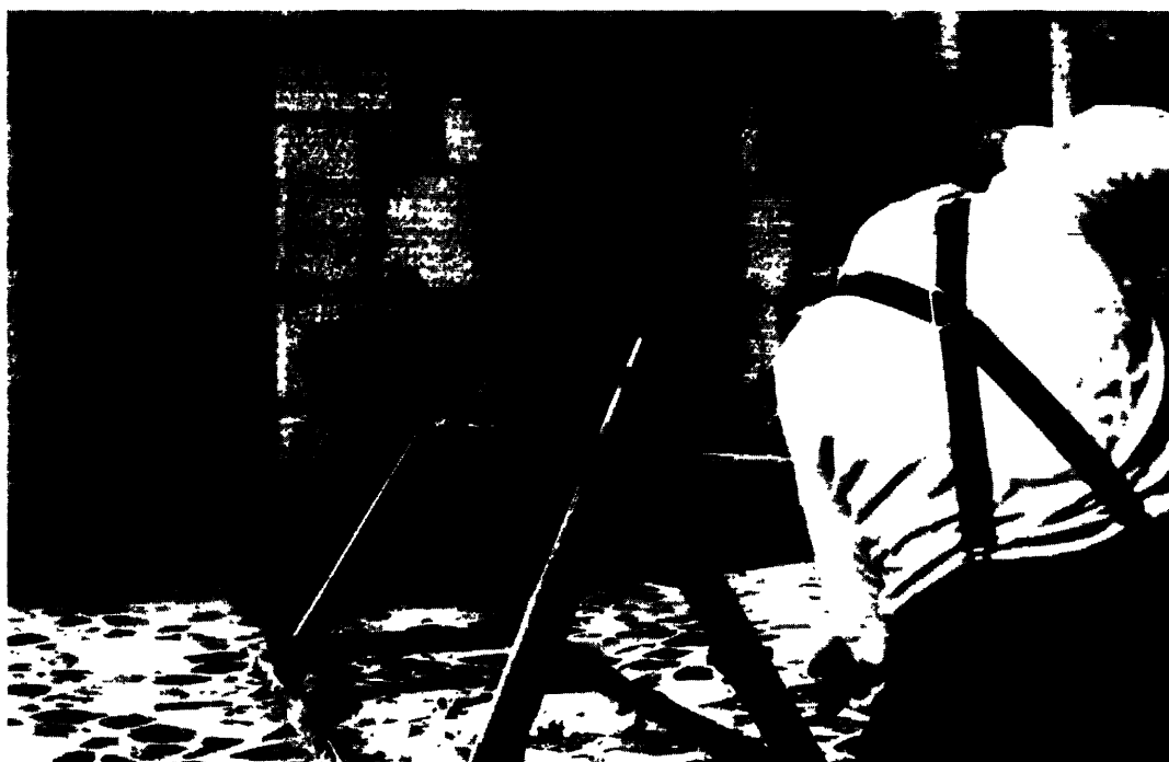
Piercing pine tree trunks to make pipes. Hand-halved pine trunks have been used to channel thermal waters since the 14th century.
