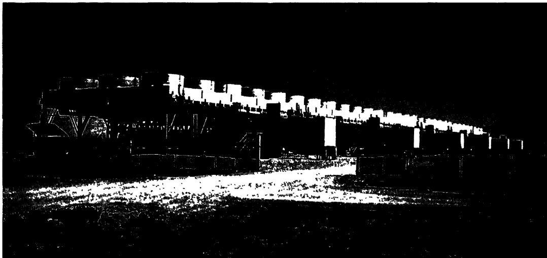
Photo - Soda Lake, Nevada 14 MW air cooled binary facility, Ormat design. Note lack of steam plume (plant was operating at time of photo), low profile, and nearby vegetation.
