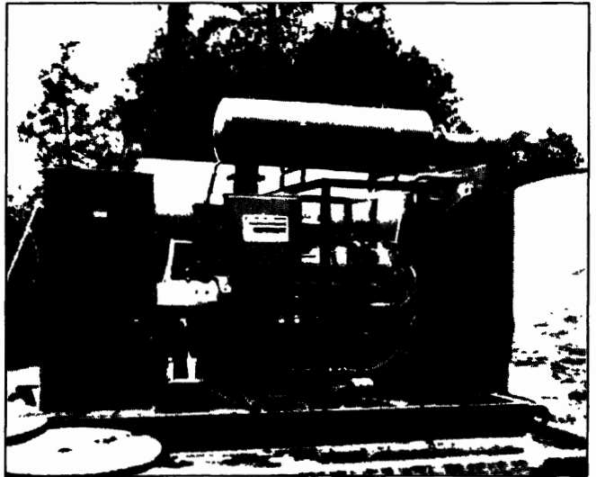
Figure 5. Emergency turbine generator.
