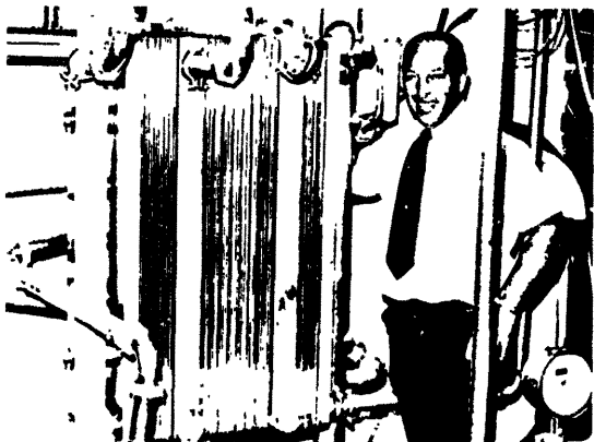
Owner, Elmer Belcastro, standing next to the plate heat exchanger (pasteurizer).
