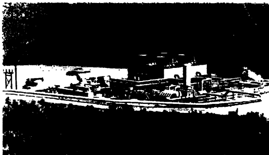
Photo 3 General View of COSO Geothermal Power Plant
