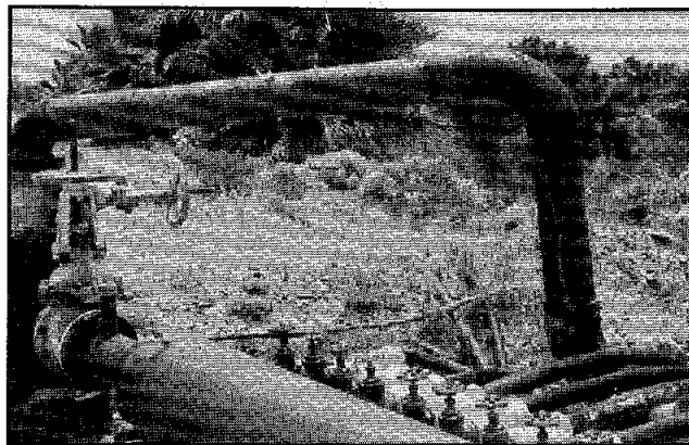
About eight, low-temperature wells are operated in the Dos Palmas Spring Area. Photo shows a well head and a manifold feed system.
