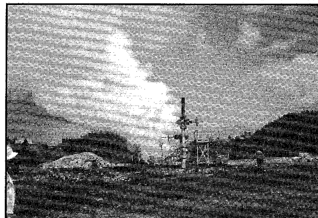
Photo 10. Kamojang Geothermal field. Well #51, drilled in June 1992, is the largest well in the field. After 3 months of testing, it will be connected to the steam plant.
