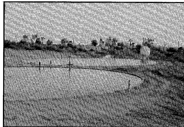
Portions of three of the four concrete fish ponds. Two ponds are 36.6 meters in diameter, and two are 30.5 meters in diameter. Photo by T. Boardman.
