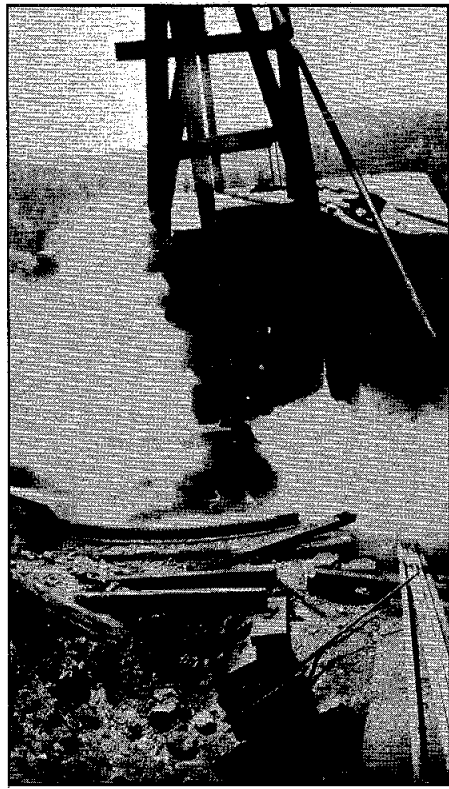
A plank across mouth of casing, weighted with drill rod weighing about a ton, fails to "hold down" steam, 1922.
