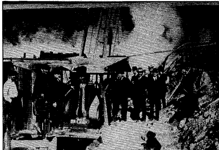
Drilling second well with steam power from first. Photo obtained from J.D. Grant.
