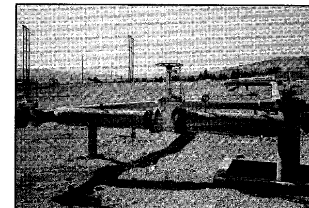
The injection well. Almost no drawdown has been measured in the reservoir.
