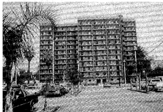
St. Bernardines Retirement Plaza, a 12-story structure included in the city's low-temperature geothermal district heating system.
