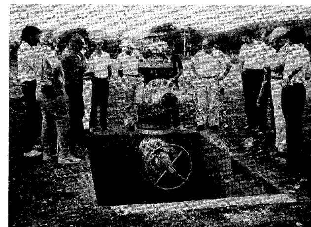
Inspecting well PGM 5R, a shallow injection test well.
