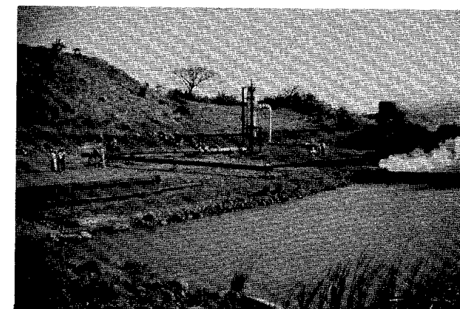
Testing well PGM 1, drilled in 1978, the first geothermal well drilled in Costa Rica.
