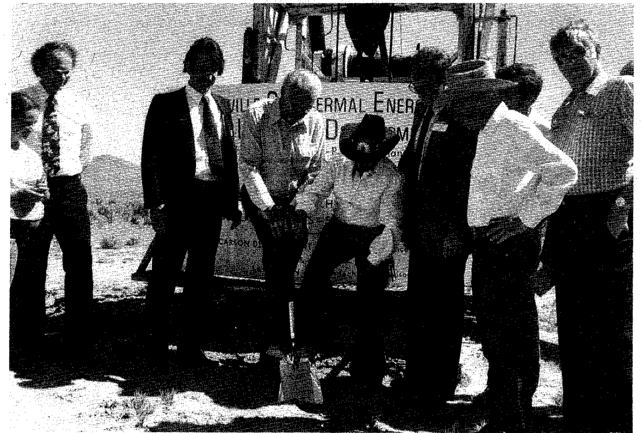
Senator Ray Johnson and Mrs. Tom Johnston break ground at the site of well "Johnston" 1, a 1500 foot geothermal well to be drilled at Litchfield, 1 1/2 miles from the Correctional Center - Susanville, and 8 miles from Susanville.
