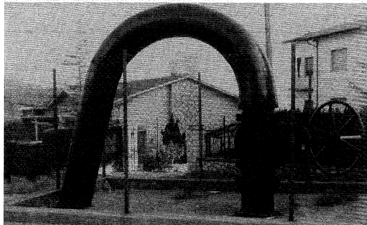
Geothermal well in Castelnuovo. Through the arc of the well pipe, and behind the house, cooling towers of the geothermal plant are visible. This geothermal reservoir has been under production for 35 years. The producing wells are between 300 meters and 500 meters deep.
