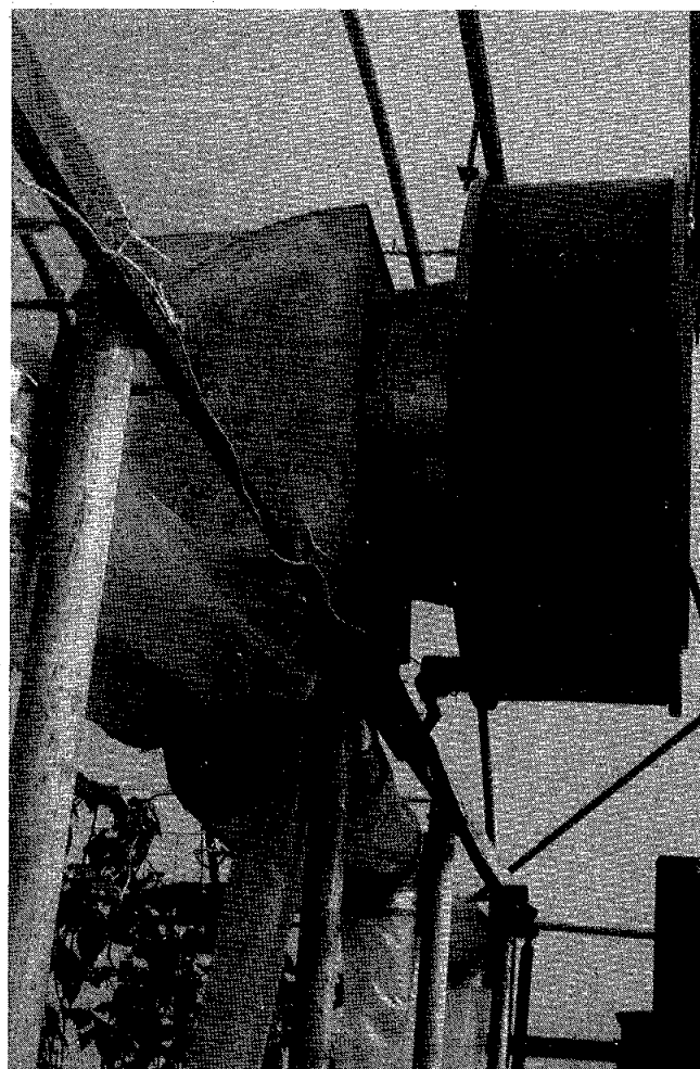
Close-up of radiator-fan unit. Air is warmed by geothermal water circulated through the radiator, and blown through the clear-plastic perforated ducts that extend through the greenhouse.
