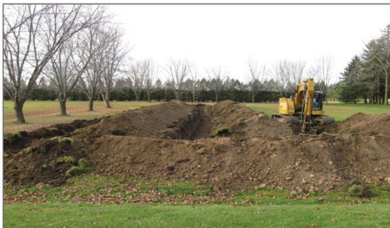
Figure 1. GLHE installation at test site in Elora, ON.
